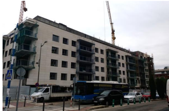
Plaza Homes (217 units) Getafe, Madrid
