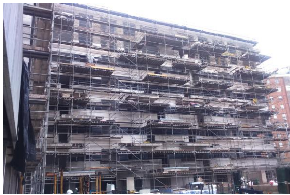
Avenida Homes (54 units). Expected delivery in H2 2018
