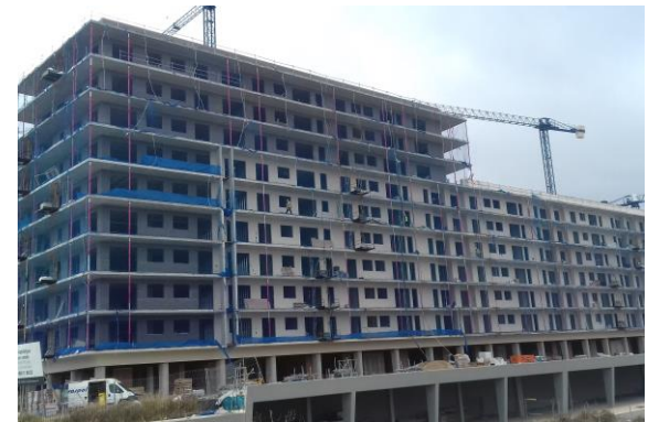
Marina de Badalona (173 units). Expected delivery in H2 2018
