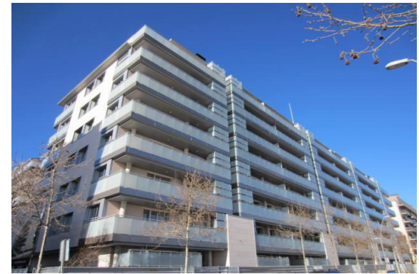
La Catalana R-4 (86 units). Expected delivery in H1 2018
