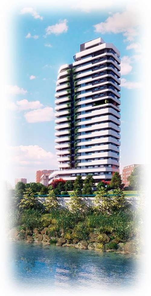
Riverside Homes – Madrid (Centro)
